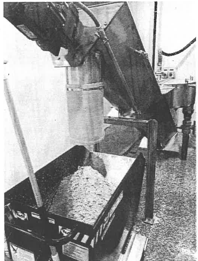
Robbinsdale's lime storage (above) and lime grit removal (below).
